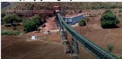
24km long pipe conveyor belt at Bellary, Vijayanagar plant
